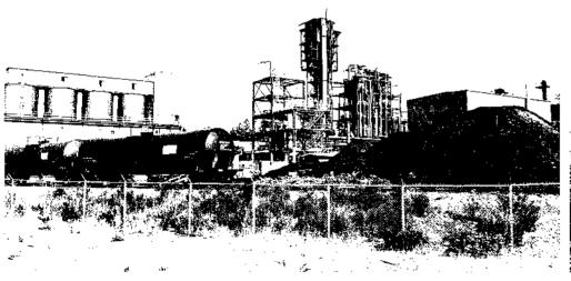
Coal pile and tank cars on a rail siding at Tacoma, Washington, symbolize the conversion of solid to liquid fuels in the 75-barrel-a-day SRC-II pilot plant operated for DOE by Gulf Mineral Resources Co.
