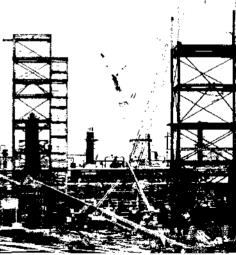
Coal bins and cranes at Catlettsburg, Kentucky, mark construction of an H-Coal pilot plant for Ashland Oil Co. The 600-barrel-a-day facility is scheduled to begin operations in 1979.
