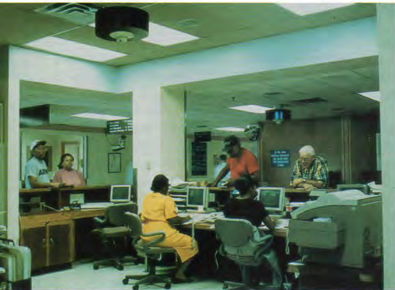
UV lamps in a hospital setting
