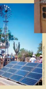
PV-powered waterpumping system in Bolivia
