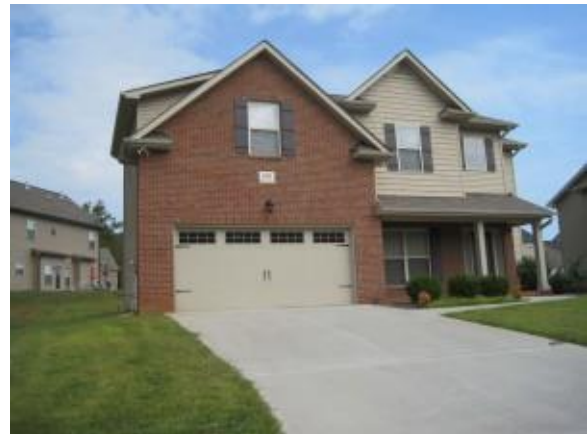
One of the experimental "robo-houses" in the energy efficiency study
