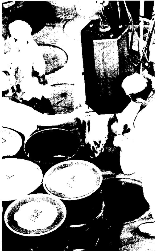
An assessment of the technological readiness of the high-temperature gas-cooled reactor has been undertaken by EPRI. Here one of the 1,482 graphite fuel blocks in the Fort St. Vrain reactor core is lowered into place. The fuel is in the small channels seen at top.
