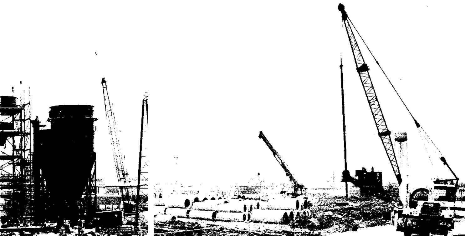
Storm drains and other site preparation at Baytown, Texas, are the early work on Carter Oil Co.'s 700-barrel-a-day EDS pilot plant, with startup scheduled for 1980. Hydrogen supply and other services will be drawn from nearby Exxon refinery.
