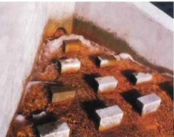
At the Springdale wetland, the leachate is pumped over a concrete aerator on its way to an equalization basin, where most of the iron removal occurs. The aerator introduces the oxygen necessary for the chemical reaction for iron removal.
