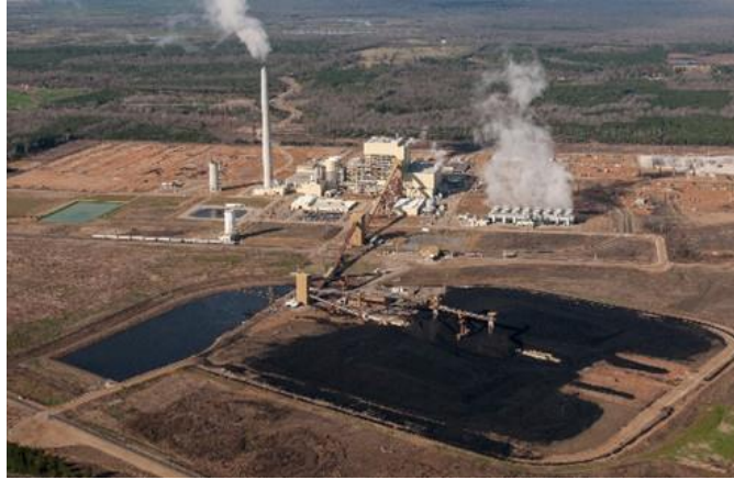
The John W. Turk, Jr. coal plant. Photo courtesy of American Electric Power.
