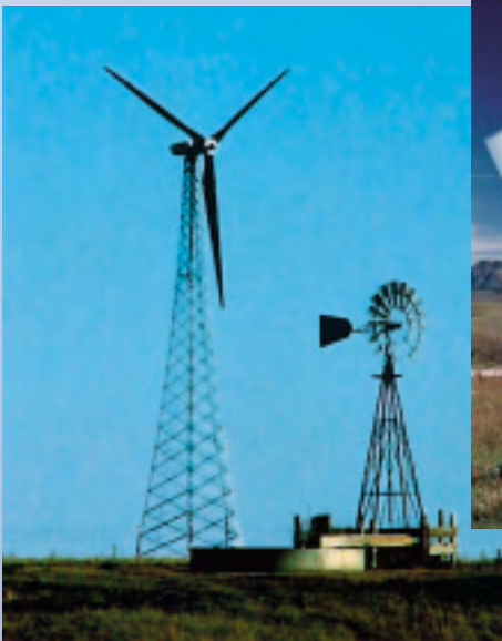
NPPD and Lincoln Electric: Springview, Nebraska; two 750-kW Zond Z-50 turbines
