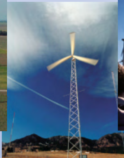
Kotzebue Electric: Kotzebue, Alaska; three Atlantic Orient 66-kW AOC 1550 turbines
