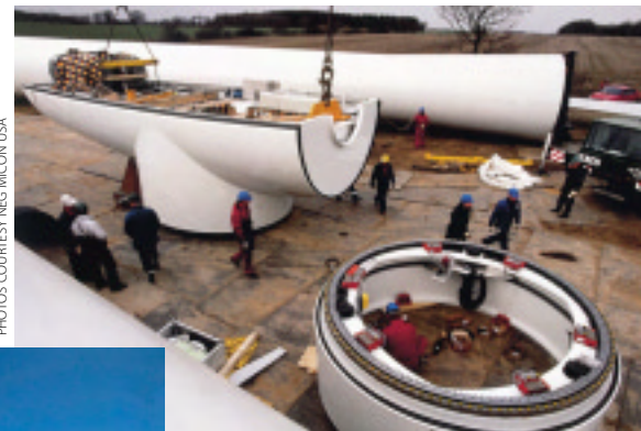
Large wind turbines and their support towers are assembled on-site with the help of very tall and expensive cranes.
