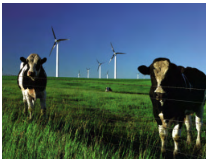
Wind farms have significant potential for economic development in rural areas because they require only small areas of land and have minimal impact on ranching and farming activities. The Zond turbines shown here are part of the 107-MW Lake Benton wind farm in Minnesota, which supplies electricity to Northern States Power.
