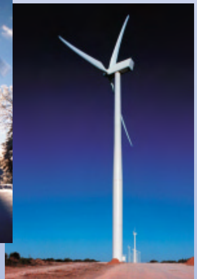
TXU Electric & Gas: Big Spring, Texas; forty-two 660-kW Vestas V47 turbines, eight 1.65-MW Vestas V66 turbines
