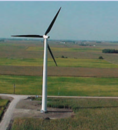
Cedar Falls Utilities: Algona, Iowa; three 750-kW Zond Z-50 turbines
