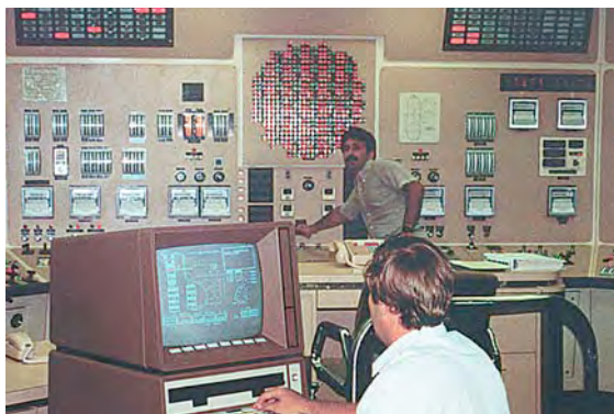
Plant control room
