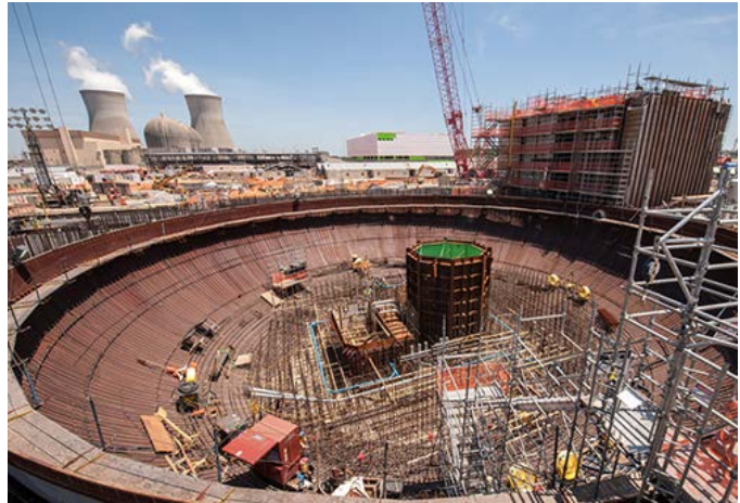
Photo of construction of Vogtle Unit 3 courtesy of Georgia Power.
