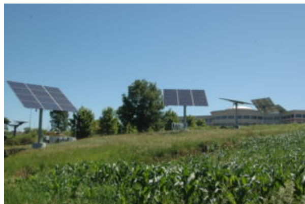
The fixed- and dual-axis tracking systems at the Madison demonstration site.
