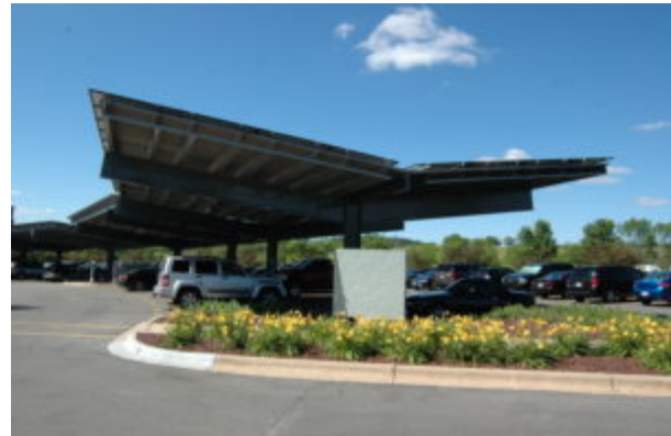
Solar parking canopies at the Madison demonstration site. Drainage is in the middle of the structures so that snow and ice do not fall on vehicles or people.
