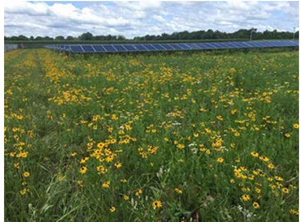
Dairyland Power Cooperative recently planted this pollinator plot at its Downsville Solar Project. Photo courtesy of Dairyland Power Cooperative.
