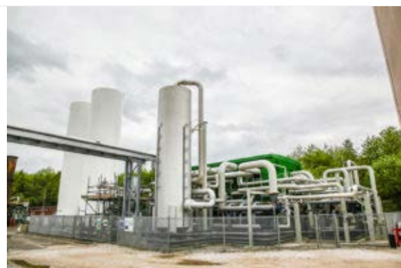
A 5-megawatt liquid air energy storage demonstration facility built by Highview Power Storage. Photo courtesy of Highview Power Storage.
