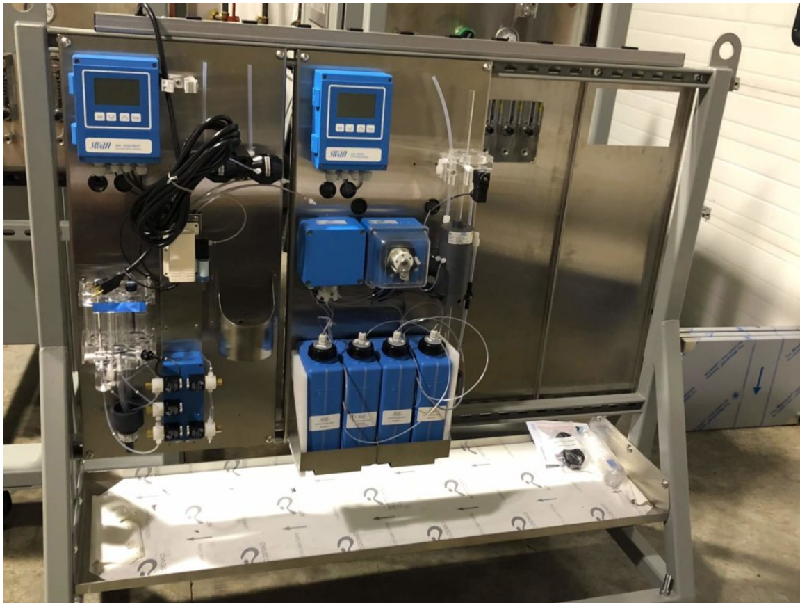
A cart of instruments for EPRI’s Smart Chemistry demonstration.
