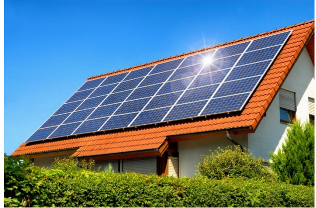
Growing rooftop solar poses cyber security challenges for the distribution grid.
