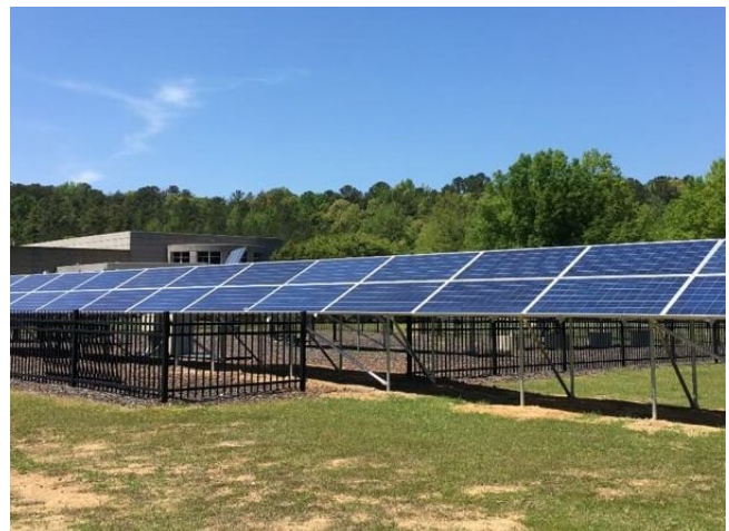
The PV modules in this array at the Southeastern Solar Research Center were subjected to accelerated aging tests before being installed outdoors. Photo courtesy of Southern Research.
