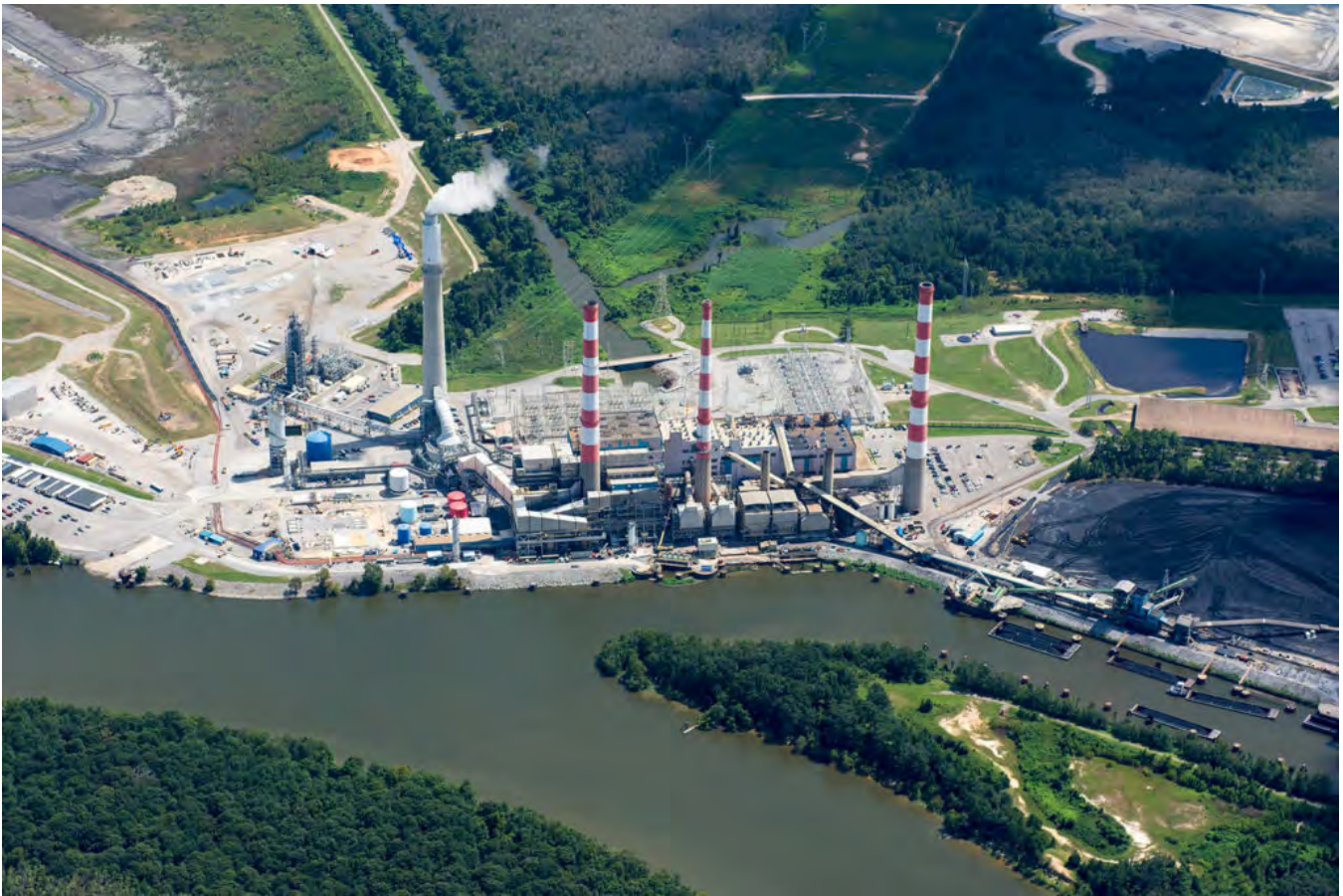
Alabama Power's James M. Barry Electric Generating Plant. Photo courtesy of Southern Company.
