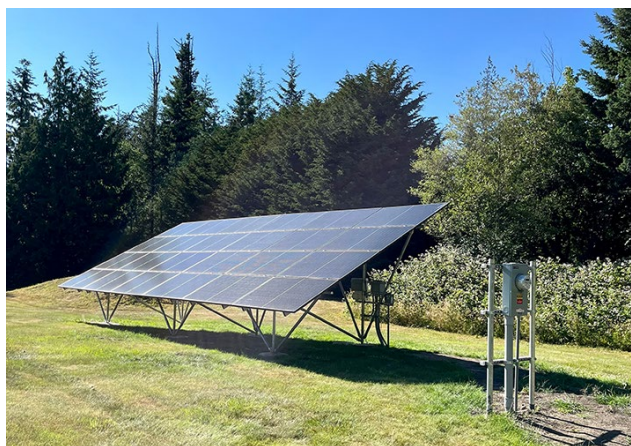
An 8-kilowatt ground mounted solar array is part of the microgrid aimed at increasing the use of clean energy within the Samish Island community.
