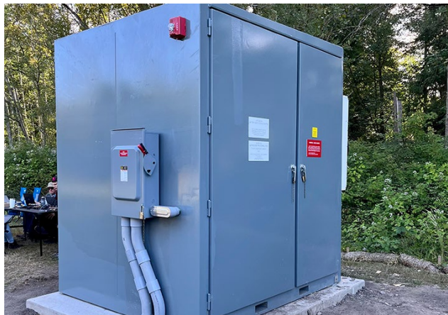
A 50 kilowatt/336 kilowatt-hour battery is part of the new Samish Island microgrid, which was installed to manage solar energy from residents on the island and provide better reliability.
