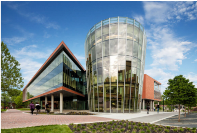
A building at Bowie State University with electrochromic windows made by SageGlass. On the right structure, the windows are in their clear state. On the left structure, some windows have darkened. Image courtesy of SageGlass.
