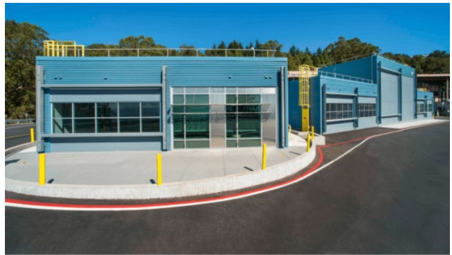
The Lawrence Berkeley National Laboratory's FLEXLAB enables users to test energy-efficient integrated building systems. In this photo, FLEXLAB is testing fixed shading and high-performance window glazings for a new Genentech office building. Photo courtesy of Lawrence Berkeley National Laboratory.
