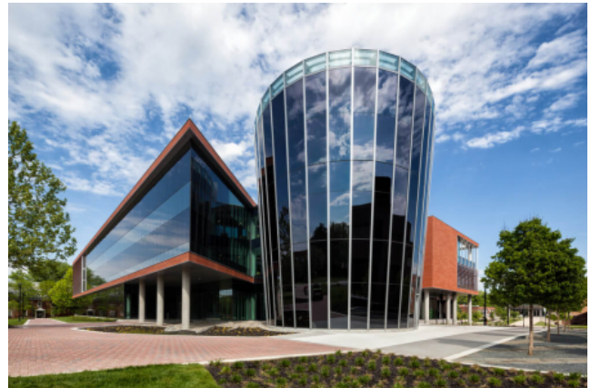
The same building at Bowie State University with most of the windows darkened. Image courtesy of SageGlass.
