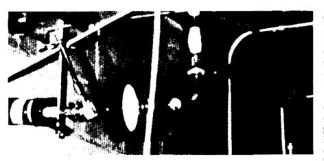
The possible release of radioactive iodine in nuclear power plants has been a major source of controversy in government regulation of the industry. EPRI has isolated prominent release points and shown how the problem can be controlled. Here a species sampler for various chemical forms of iodine is sampling the in-plant ventilation air from a BWR ceiling duct.
