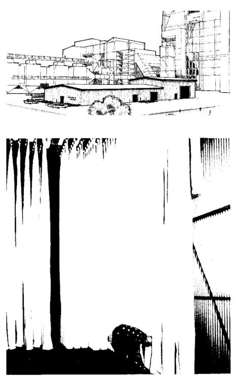
Fabric filters are efficient for particulate removal from stack gases, but many are required. For reliability in a large installation ( $\sim$ 500 MW), the baghouse may be divided into 30–50 compartments like this one, each containing 200–600 bags.
