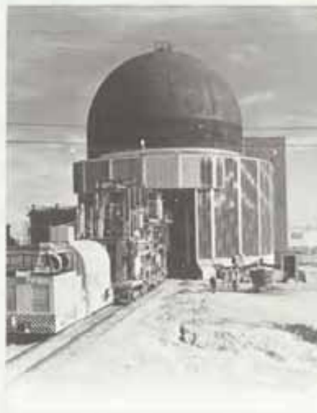
The mobile LOFT reactor shown entering its "home" with the aid of a switching engine. The facility is designed for maximum flexibility in experiments to verify safety.
