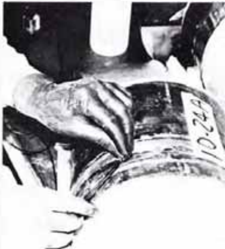
Figure 4 A typical 180° section test sample of 10-in core spray line.
