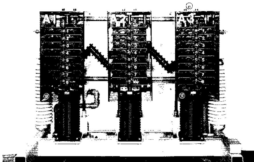
**Figure 2** Thyristor switch assembly that will control current through 13.8-kV shunt reactors of the static VAR generator to be installed on the Minnesota Power & Light Co. system.
