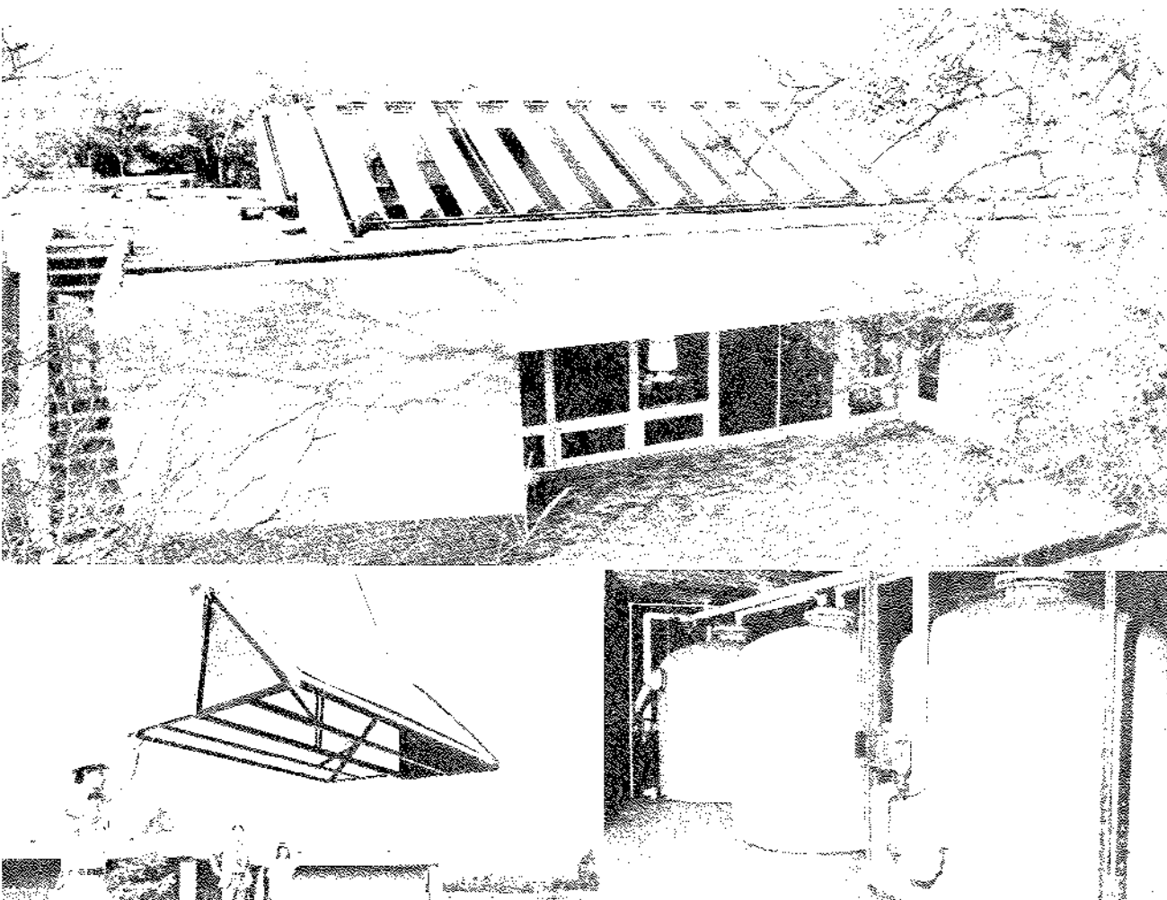
Across the country: Arlington, Texas, house (top) features a comparison of solar-absorption and vapor-compression cooling systems. Huntington Beach, California, office (left) has 15 cubic meters (4000 gal) of water to store either solar heat or rejected heat pumped from inside the building. Naylor, Maryland, house (right) uses three 3.5-cubic-meter (900 gal) insulated fiberglass tanks of solar-heated water to supplement a heat pump for year-round forced-air heating and cooling.
