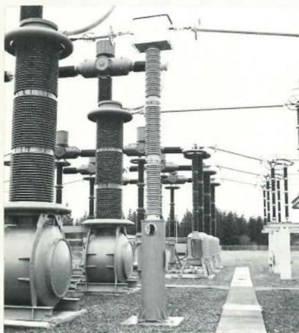
Figure 7 Prototype 500-kV electronic current transducer now installed in Bonneville Power Administration's Ostrander Substation for a one-year field trial of its digital-optical conversion and signal transmission system.
