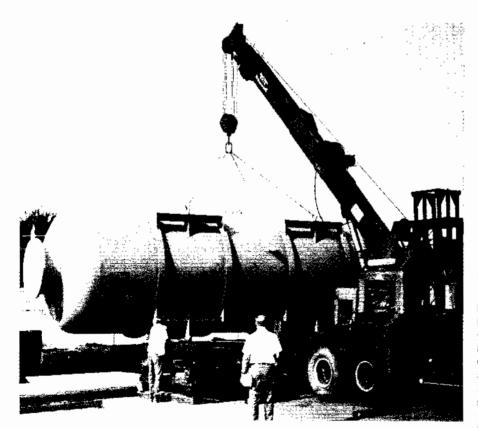
Figure 5 Prototype compact capacitor tank being off-loaded at Gould's Greensburg, Pennsylvania, facility for testing. This tank houses a 345-kV, 24-MVAR capacitor bank intended for installation on Consolidated Edison's system in New York.
