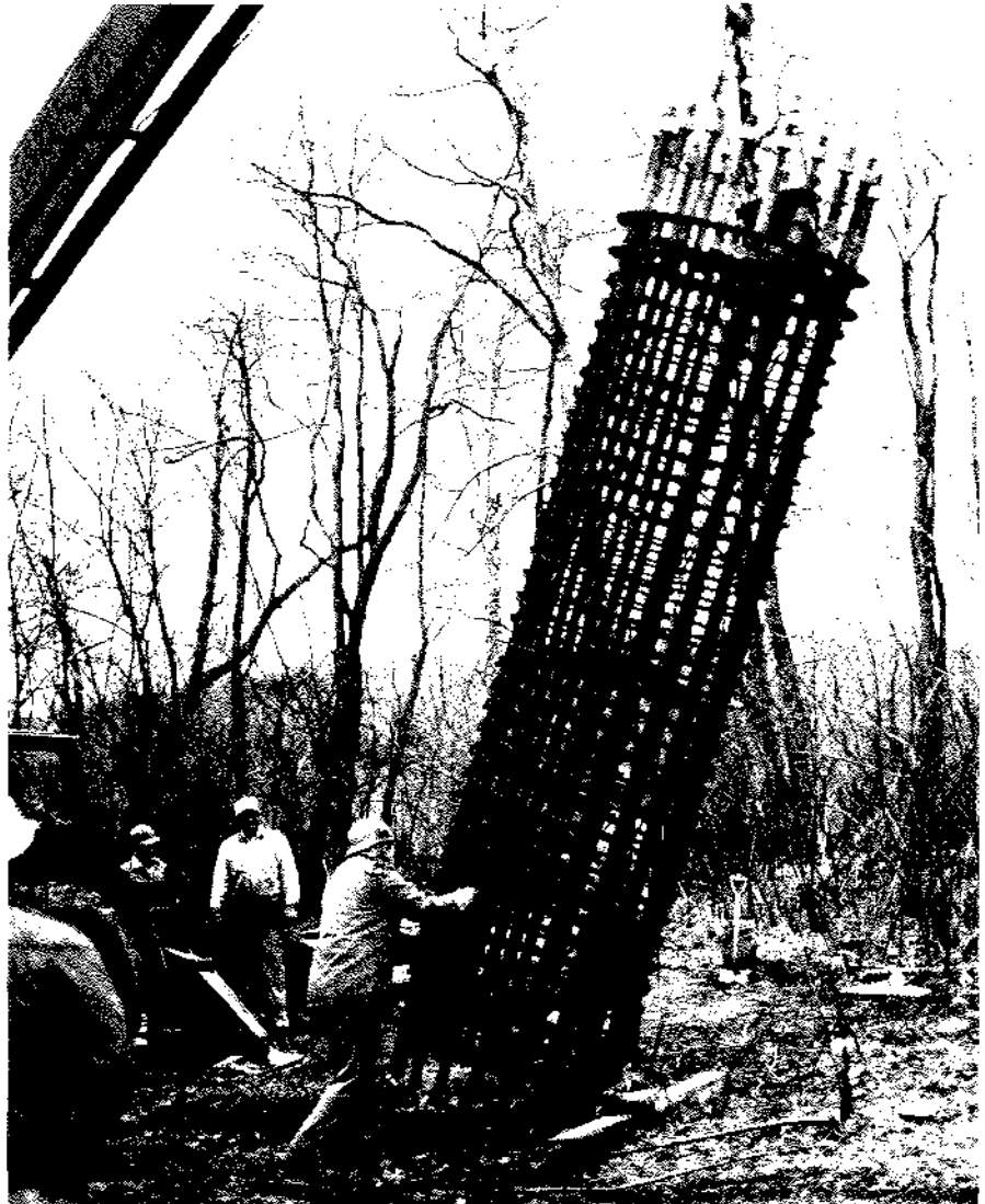
Figure 1 Construction of a typical pier for transmission line towers consists of augering a hole, inserting an anchor bolt cage, and backfilling the hole with concrete. This particular cage is 14 ft long and weighs more than 5000 lb.
