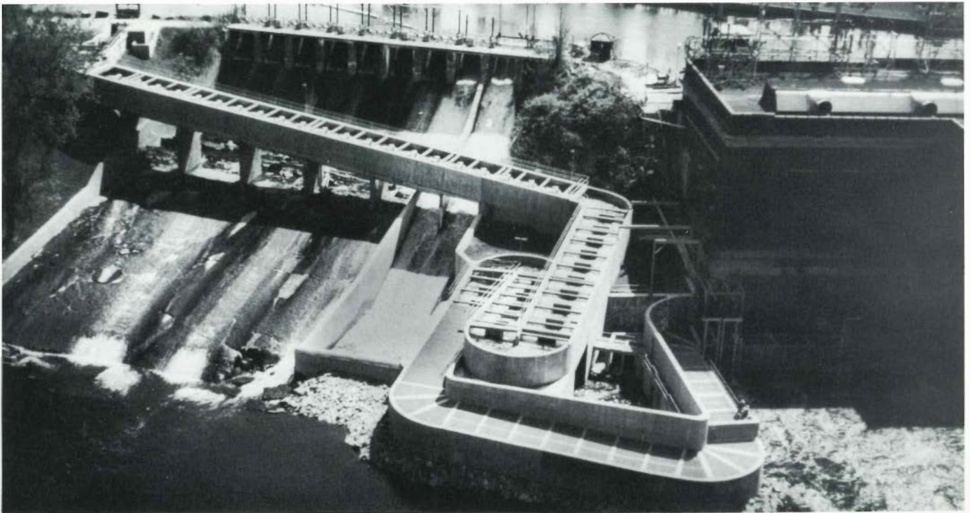
Where hydroelectric power plant dams are barriers to fish migration, fish ladders and elevators are providing the necessary bypass for the fish to move upstream. This fish ladder is at Western Massachusetts Electric Co.'s Turners Falls plant on the Connecticut River.
