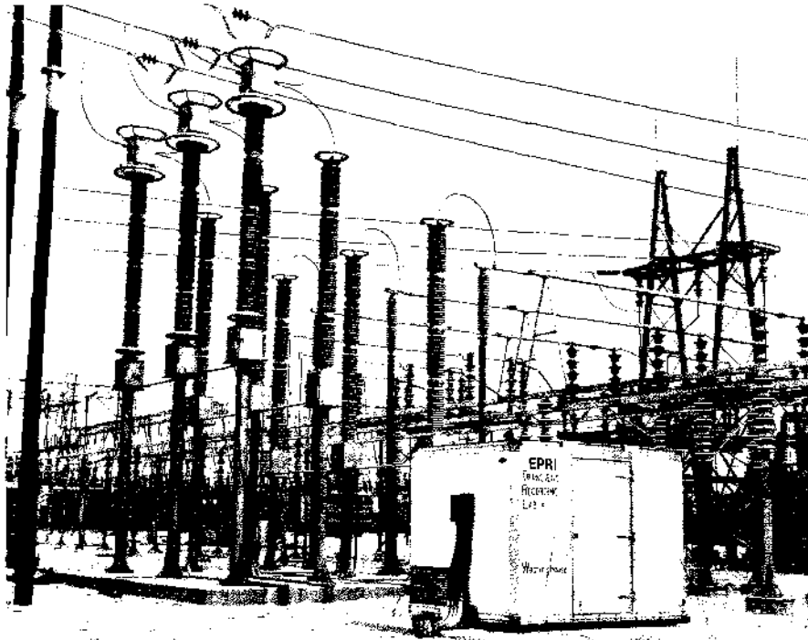
Figure 2 Instrumentation system installed at Florida Power & Light Co.'s Lauderdale substation for detection and recording of switching surges.
