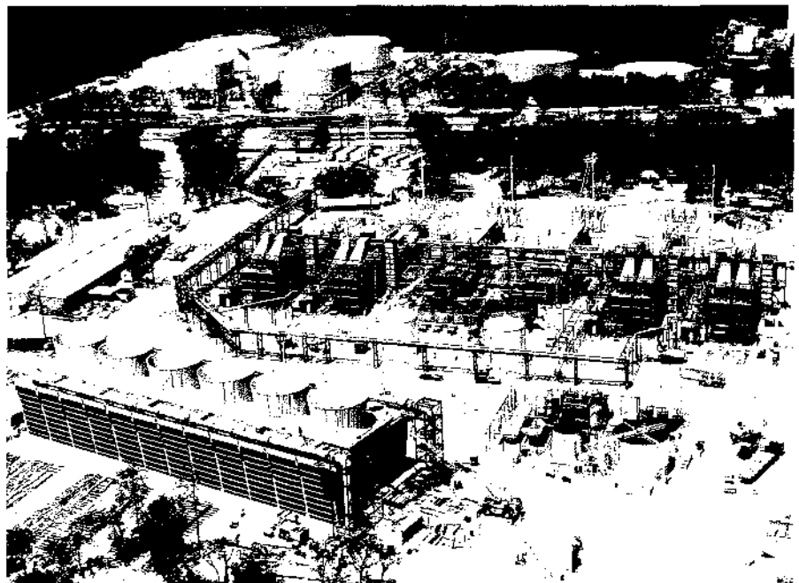
Figure 1 Tests were conducted at Florida Power & Light Co.'s Putnam station to determine the operating cost differential between light and heavy oil.
