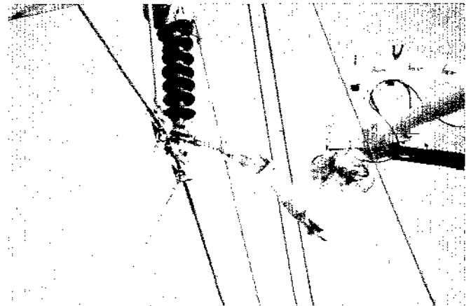
Figure 1 Remote-controlled line maintenance device. (a) To demonstrate the concept of using such a device, the bucket on a Pitman boom truck was replaced with a General Electric manipulator. With this setup and a closed-circuit TV system, a string of insulators was replaced by operating controls mounted in the truck bed. (b) Close-up of the manipulator.
