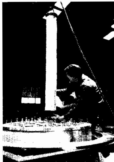
Figure 1 A 3M Co. alumina-bore-silica bag is lowered into the Buell fabric filter assembly at Westinghouse's Waltz Mill facility.
