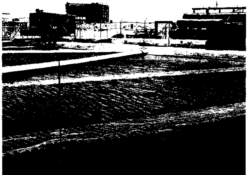
Solar salt ponds operate on a principle similar to that of OTEC. The sun's heat passes through the top, freshwater layer of the pond and concentrates in the lower, salty layer. Ormat Turbines of Israel has operated test ponds for several years.
