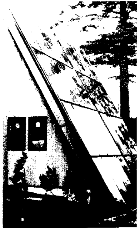
Active SHAC systems use mechanical devices to collect, store, and distribute the sun's energy. The main components of an active system include solar collectors, pipes, pumps, and fans.
