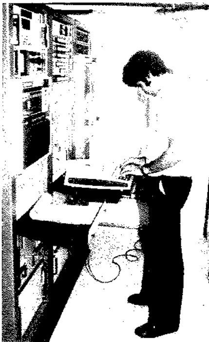
Figure 1 Interior of the mobile trailer that houses the real-time digital data acquisition system. Using the computer equipment shown, test data can be safely and accurately recorded in substations up to 765 kV.
