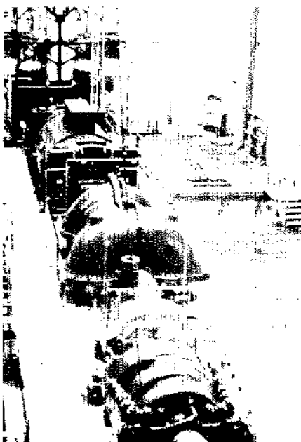
Figure 1 Turbomachinery of the 290-MW (50-Hz) salt-dome CAES plant in Huntorf, Federal Republic of Germany. The success of this plant has provided the major impetus for efforts to commercialize a similar system in the United States.
