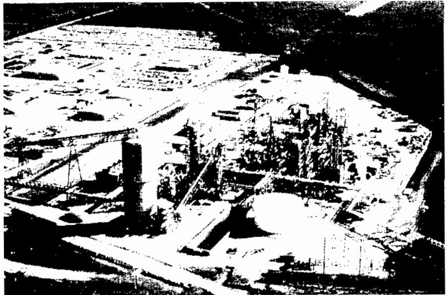
Figure 1 The Exxon coal liquefaction pilot plant at Baytown, Texas.
