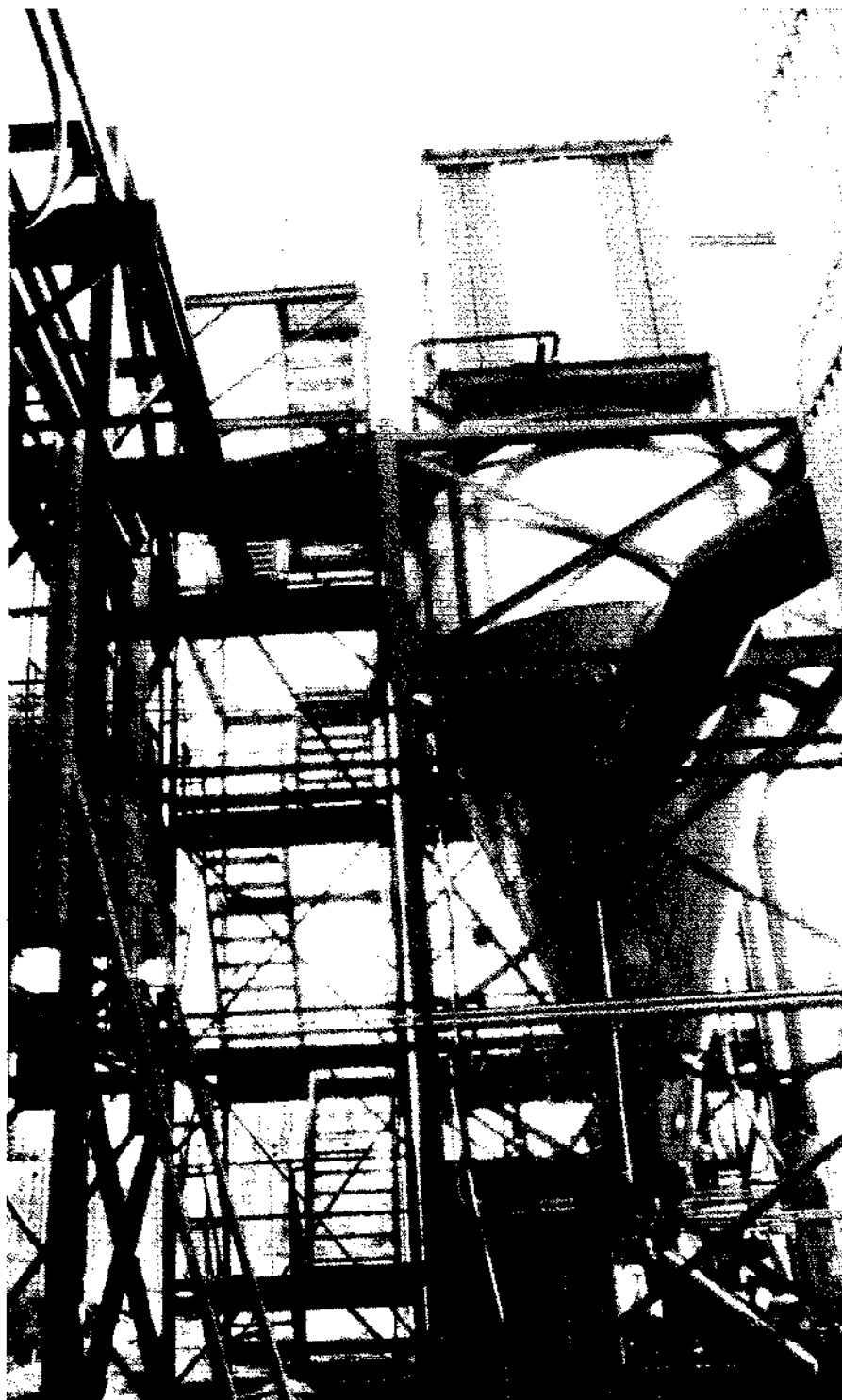
Figure 3 The 2.5-MW spray drying FGD pilot unit at EPRI's Arapahoe test facility.
