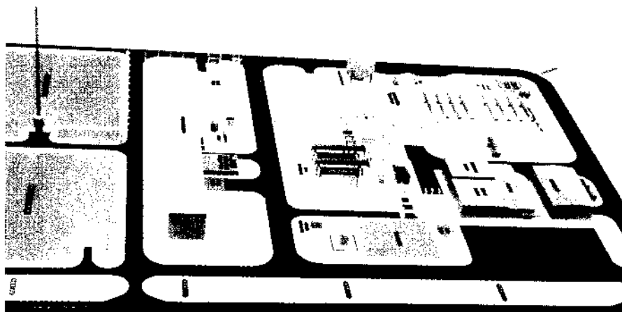
Figure 2 The model of the Heber binary-cycle plant that will be used for construction is already taking shape at the facilities of Fluor Engineers and Constructors, Inc., in Irvine, California. The model will be transported to the site to support construction in mid 1983.
