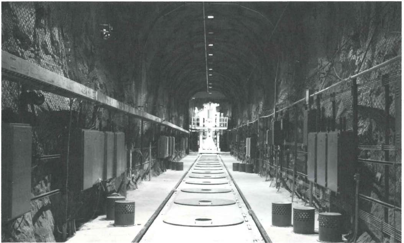
At the Climax Mine at the DOE's Nevada Test Site, 1400 feet below the surface, 11 spent fuel bundles have been buried to permit measurement of thermal and radiation effects of waste disposal in granite. This facility is the first demonstration of emplacement of significant quantities of spent fuel in a geologic media in the United States. Results from the demonstration will be helpful in designing permanent disposal facilities for vitrified high-level waste.
