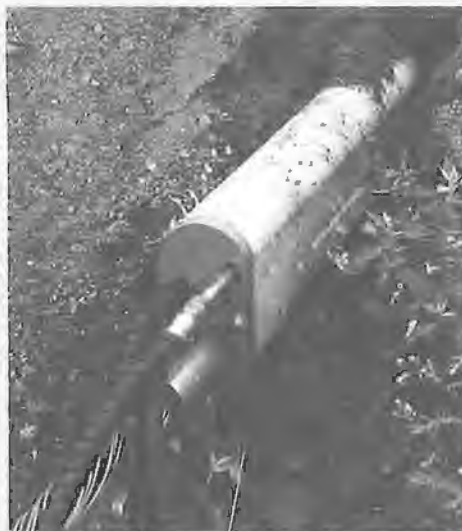
Figure 4 Cable follower loaded onto a cable and entering the ground at the end of a failed cable. The water and hydraulic fluid are now entrained in a single umbilical cord.
