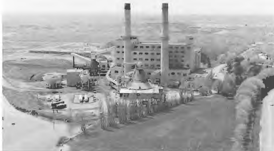
There are dozens of MSW-to-energy recovery programs across the country, from RDF cofiring in Ames, Iowa, and Rochester, New York, to dedicated MSW-burning boilers in Nashville and Gallatin, Tennessee, to landfill gas recovery in Mountain View, California.
