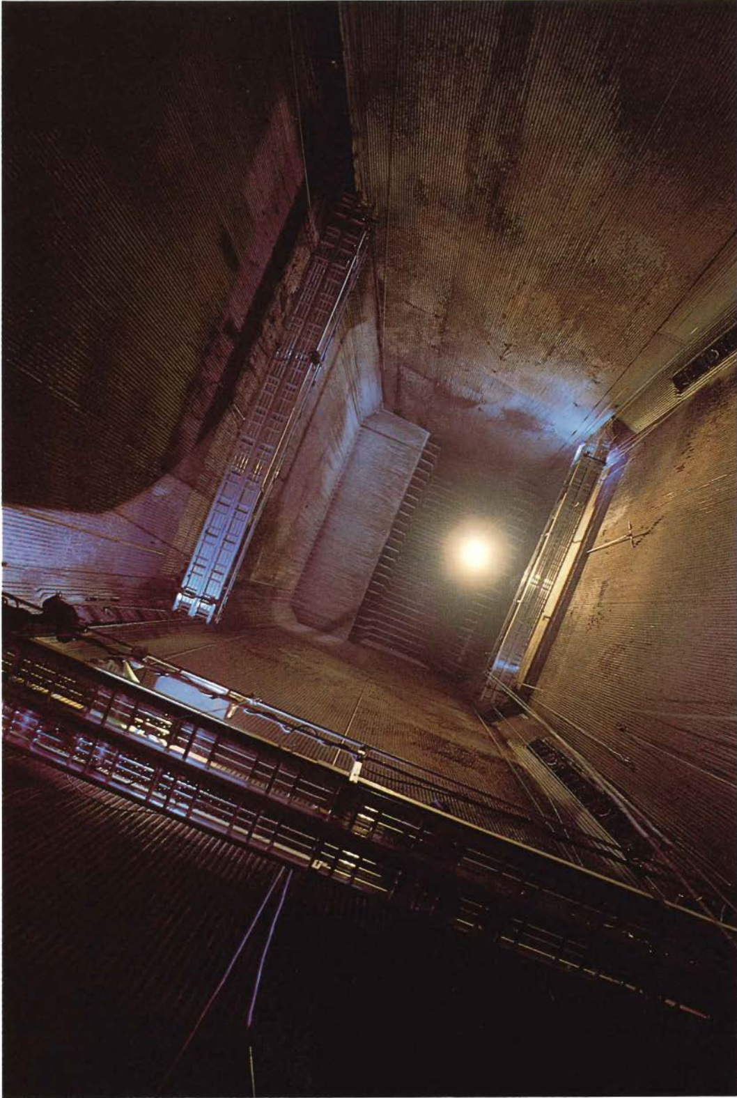
View from the bottom of a coal-fired boiler.
