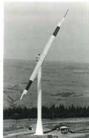
Wind turbines are being proved today in sizes up to 2.5 MW. Clusters of such machines can produce supplemental electricity without fuel cost.
