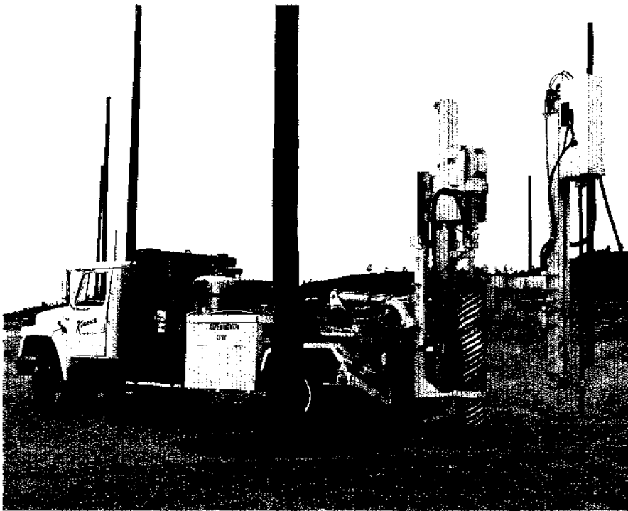
Figure 3 With a new ground-line pole-repairing (stubbing) technique, standard industrial augering equipment with vibratory torque-multiplying action can be used to screw a section of helical tubing (culvert) into the ground around a pole butt in less than one minute. The pole at left has already been repaired, and the annulus between the pole and the steel tube was filled with a resin that cures to a strength several times that of concrete; the resin also contains a time-release fumigant to prevent further decay under the repair section.
