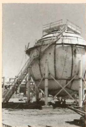
The 44-ft-diam (13.4-m) carbon steel hydrocarbon storage sphere can hold the entire hydrocarbon inventory when the plant is not operating. When the plant is running, the sphere is about 10% full.
