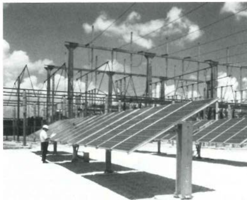
FP&L's 10-kW flat-plate array in Miami
