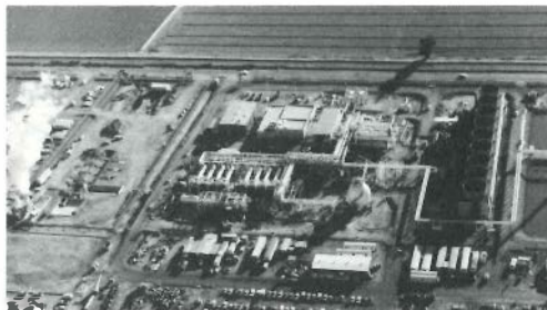
Heber geothermal plant
