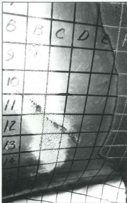
Figure 2 Evaluation grids like this one are used on turbine runner blades in order to compare cavitation pitting from inspection to inspection. Here the cavitation damage appears as the rough, lighter area near the center of the shiny stainless steel overlay.
