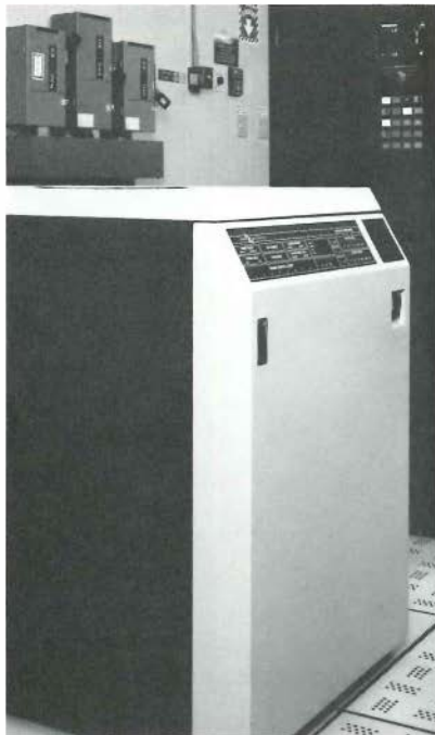
Power line conditioner
