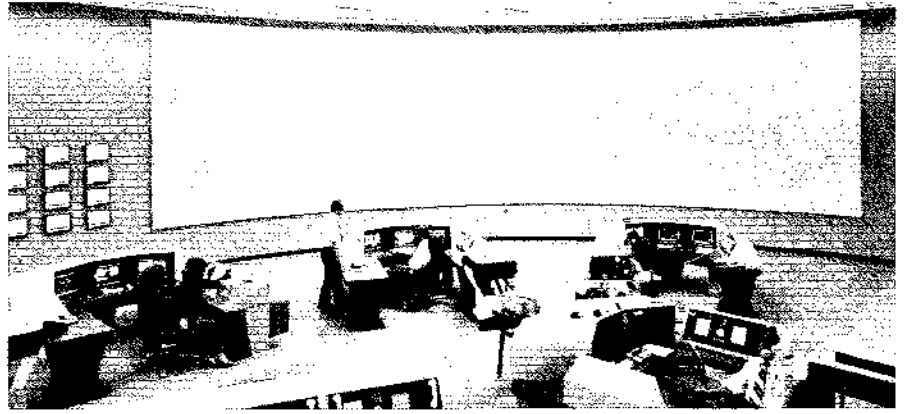
Florida Power Corp. control room
