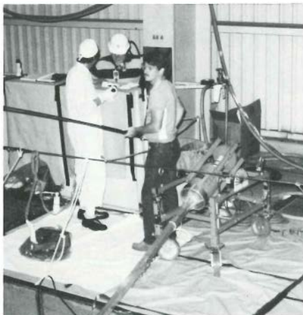
Assay of irradiated hardware under water.
