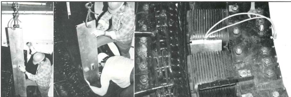
Generator with scanner in place
