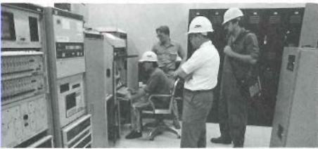
Acoustic leak monitor and vibration analyzer
