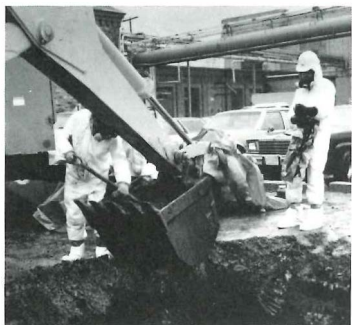
▲ Source removal by excavation
