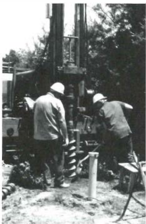
▲ Groundwater well drilling
