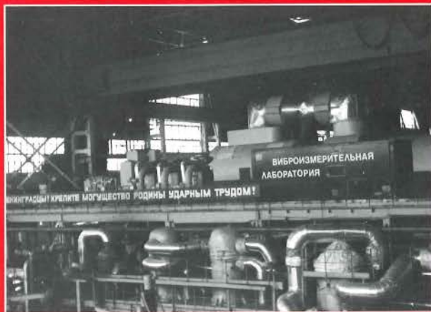
In-plant testing of new technology, a common Soviet practice, is seen in this turbine-vibration-monitoring trailer at Leningrad's Southern station; the slogan reads "Work hard for the common good."
